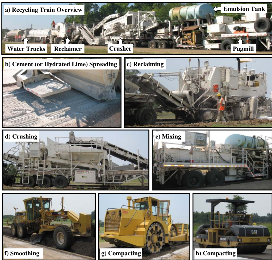
Figure 6.3 US-49 CIR Construction Photos
